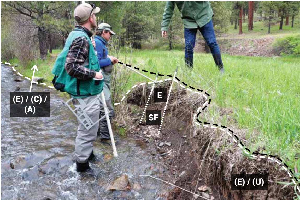
Figure H.11. The water surface is at the scour line in this photo. The bank in the background is erosional (E), covered (C), and absent (A). The bank in the foreground is erosional (E) and uncovered (U). The upper part of the bank is nearly vertical and eroding (E), while the lower part of the bank has an accumulation of slough (SF). It is not uncommon to have more than one instability feature in the streambank stability quadrat. In this case, the instability feature could be listed as either eroding (E) or slough (SF).
