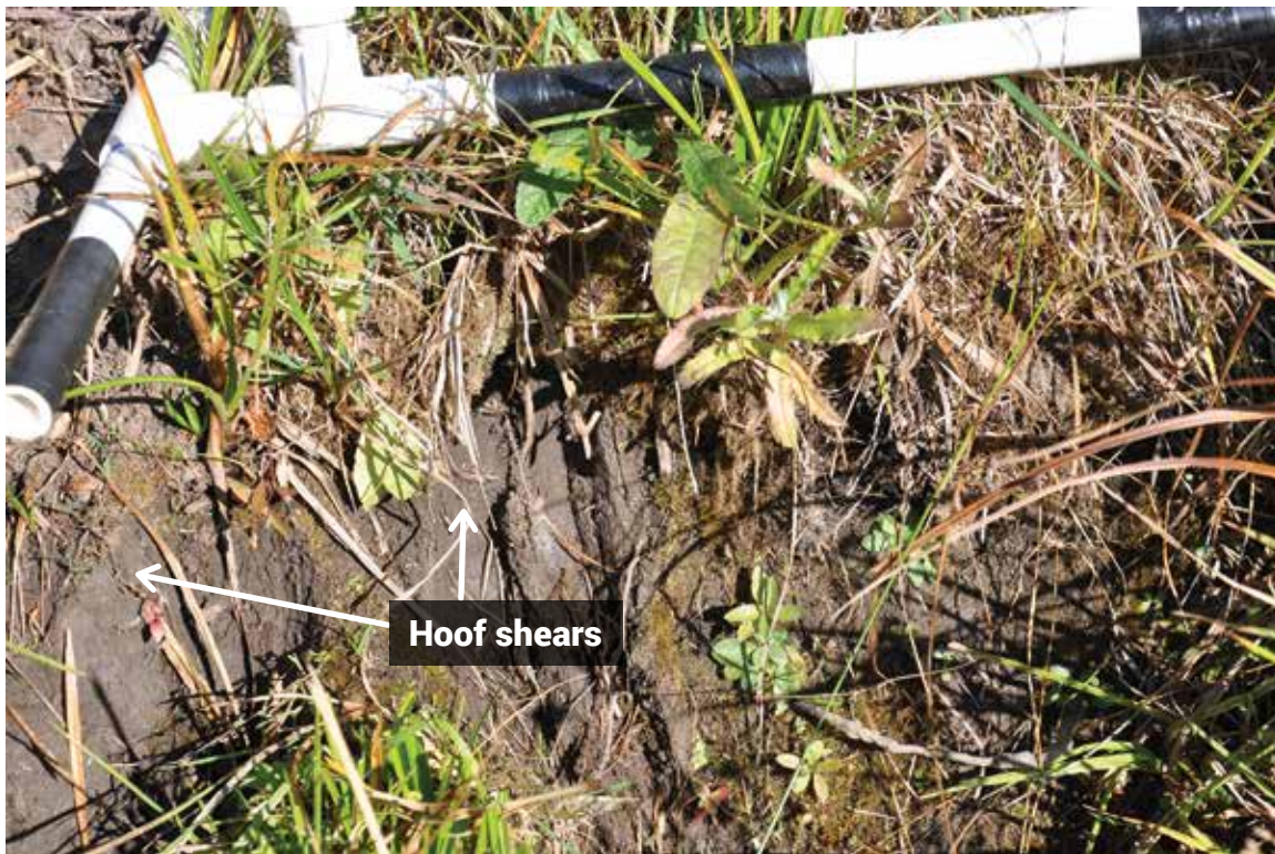
Figure E.7. Close up view of hoof shears on vertical face of bank. Notice the “tooled” look to the soil face.
