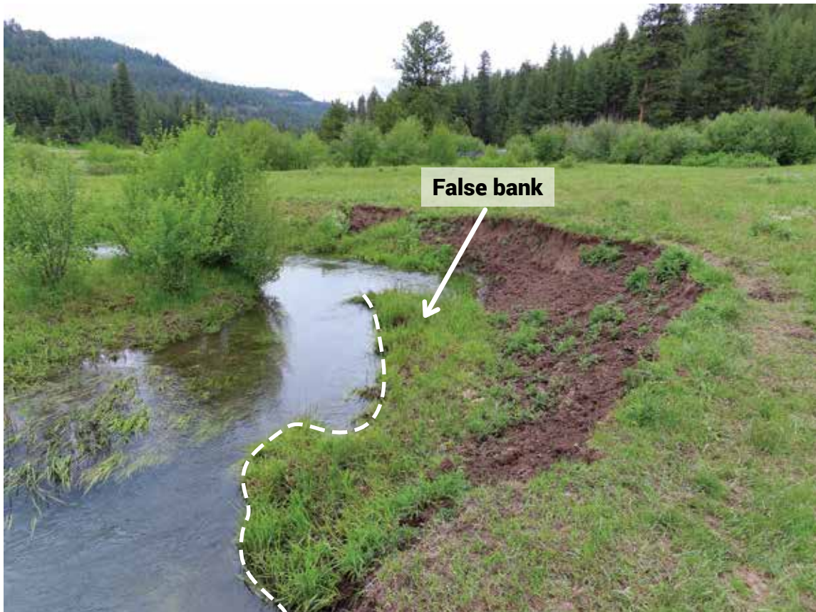
Figure D.30. Some false banks are subject to annual trailing/trampling impacts behind them; as a result, they may be sloped back to the edge of the terrace with considerable bare ground. If there are no fracture features or stream erosion behind them, they are stable and not considered slump blocks. The greenline is at the edge of the vegetation above the water's edge where the greenline rules have been met.
