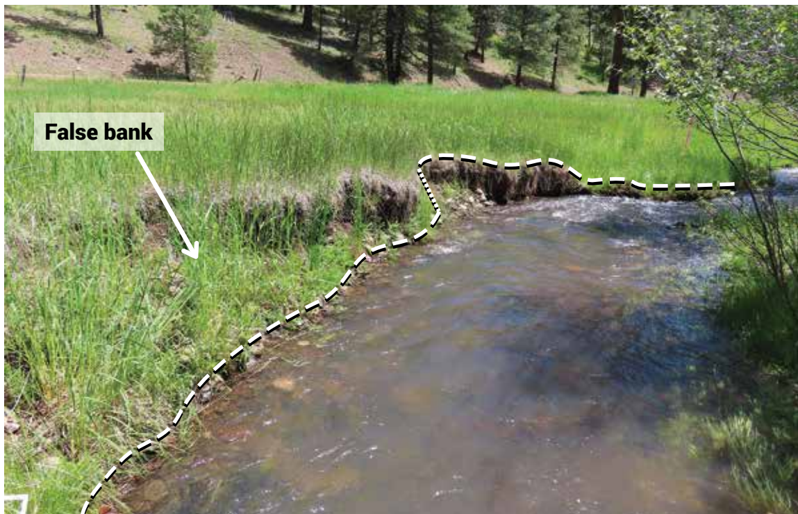
Figure D.29. False banks are sections of bank (slump blocks) that have broken off from a high bank or terrace and have become reattached. They may also be places where slough material has accumulated at the base of terrace walls and has become vegetated. This false bank (see arrow) is vegetated back to the terrace wall, there is no fracture or erosion behind it, and it is a stable feature. The greenline follows the water's edge where the greenline rules are met.
