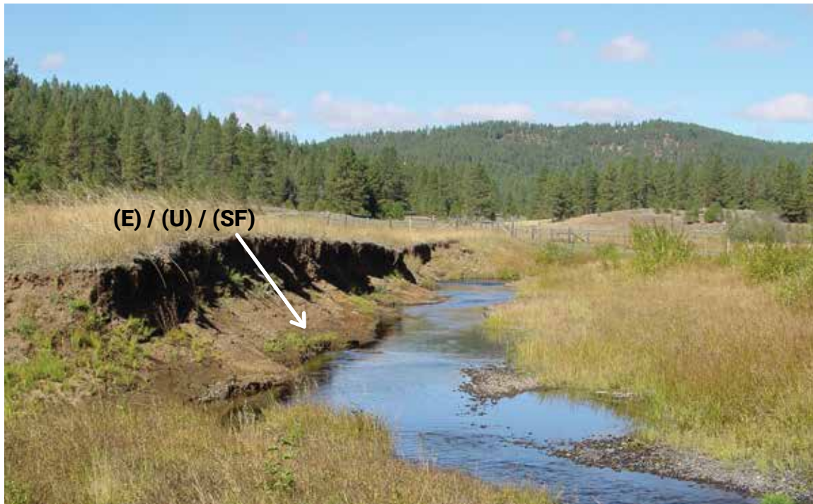
Figure H.9. The left bank in this photo is erosional (E) and uncovered (C) with no vegetation, rock, or wood. The lower two-thirds of the bank has accumulated loose aggregates of soil, or slough (SF), which likely will be removed from the bank during high streamflow.
